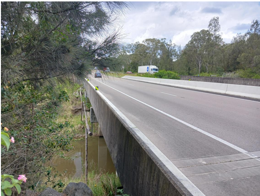
Image 4: Balickera Canal Bridge to be widened
