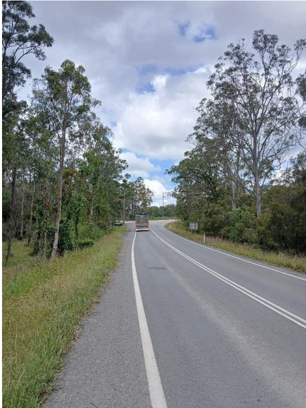
Image 1: Limit of road works – Italia Road
