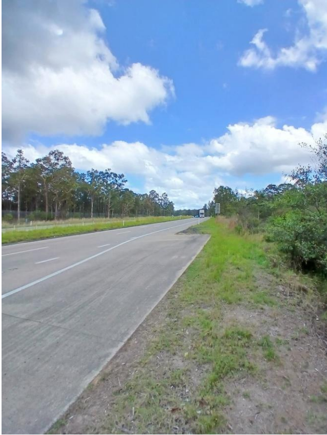
Image 3: Limit of north bound Pacific Highway roadworks
